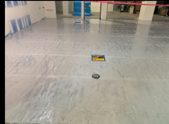
Floor Prep for Terrazzo
