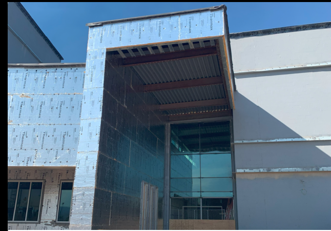
Exterior Glazing and Insulation
